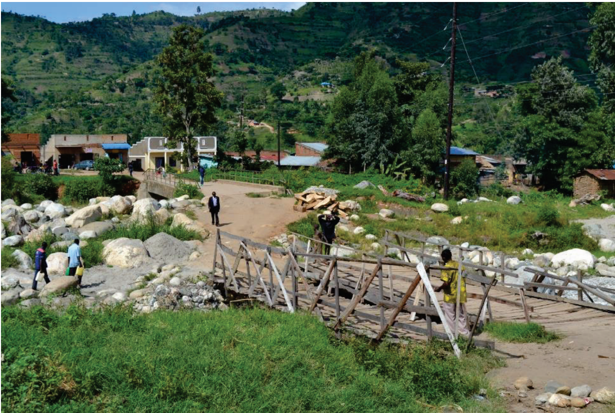
Figure 10. The original bridge in the background, and a bridge constructed following the floods in the foreground, in Kasese District, Uganda. Residents cope with extreme events by increasing riparian buffers and resettling to higher ground.
